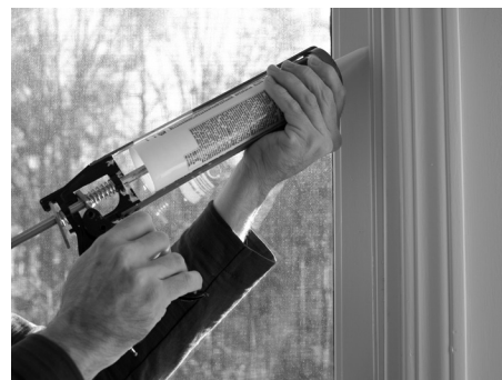
▲ Sealing air leaks in your home can help you save on heating and cooling bills. (Image credit: Alyson Hurt)
