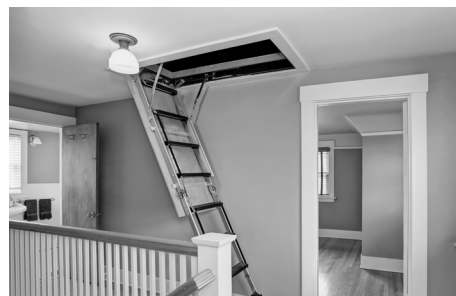
▲ Even a well-insulated attic can leak air through the stair opening. An insulated cover box can seal and insulate this opening.
